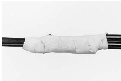
**5** Construct joint according to standard procedure and wrap joint with insulating material (not included in standard kit).
