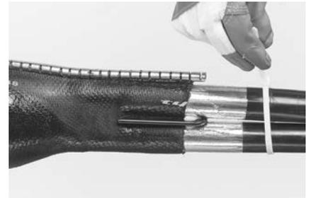
**21** For branched joints only: press the cables together with a tie wrap from the BOKT-kit.
