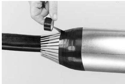
**8** Using PVC-tape (not included in standard kit), tape the crowns, starting from the canister body, down to the cable.
