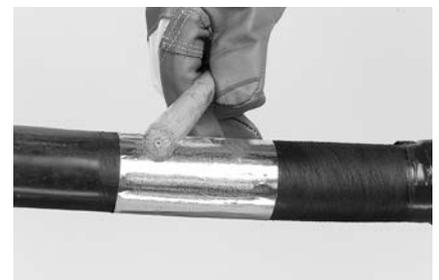
**12** Smooth the aluminium tape with a blunt tool to smooth sharp edges.
