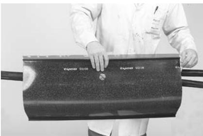
**10** Center the sleeve over the canister by placing the metal ring in the sleeve over the valve in the canister. Mark ends of sleeve on cable jacket.
