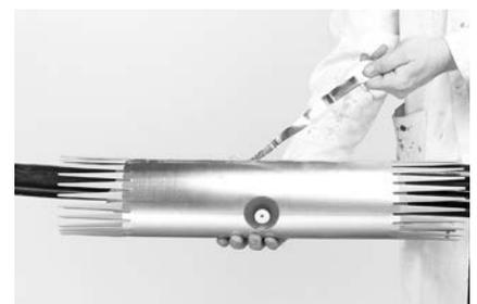
**6** All sizes: assemble the two half shells symmetrical to form a hinged canister and secure one of the seams with self-adhering aluminium tape. Center and fit metal canister over the joint. Smooth the tape with a blunt tool.
