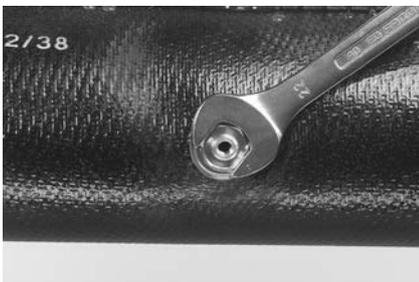
**25** Allow the sleeve to cool down undisturbed for at least 15 minutes. Tighten the valve nut.
