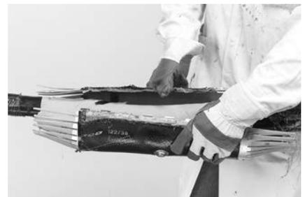
**9** Remove the canister and rework the splice.
